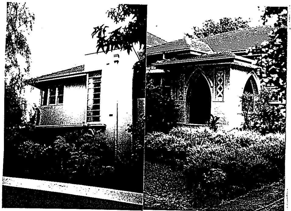
3.60 Glen Eira Road houses, including the tower of "Nithsdale", glimpsed from Glen Eira Road.
