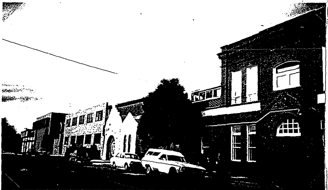
Selwyn Street showing the former Elsternwick Fire Brigade building (1895-1926) and recent commercial development to the north.
