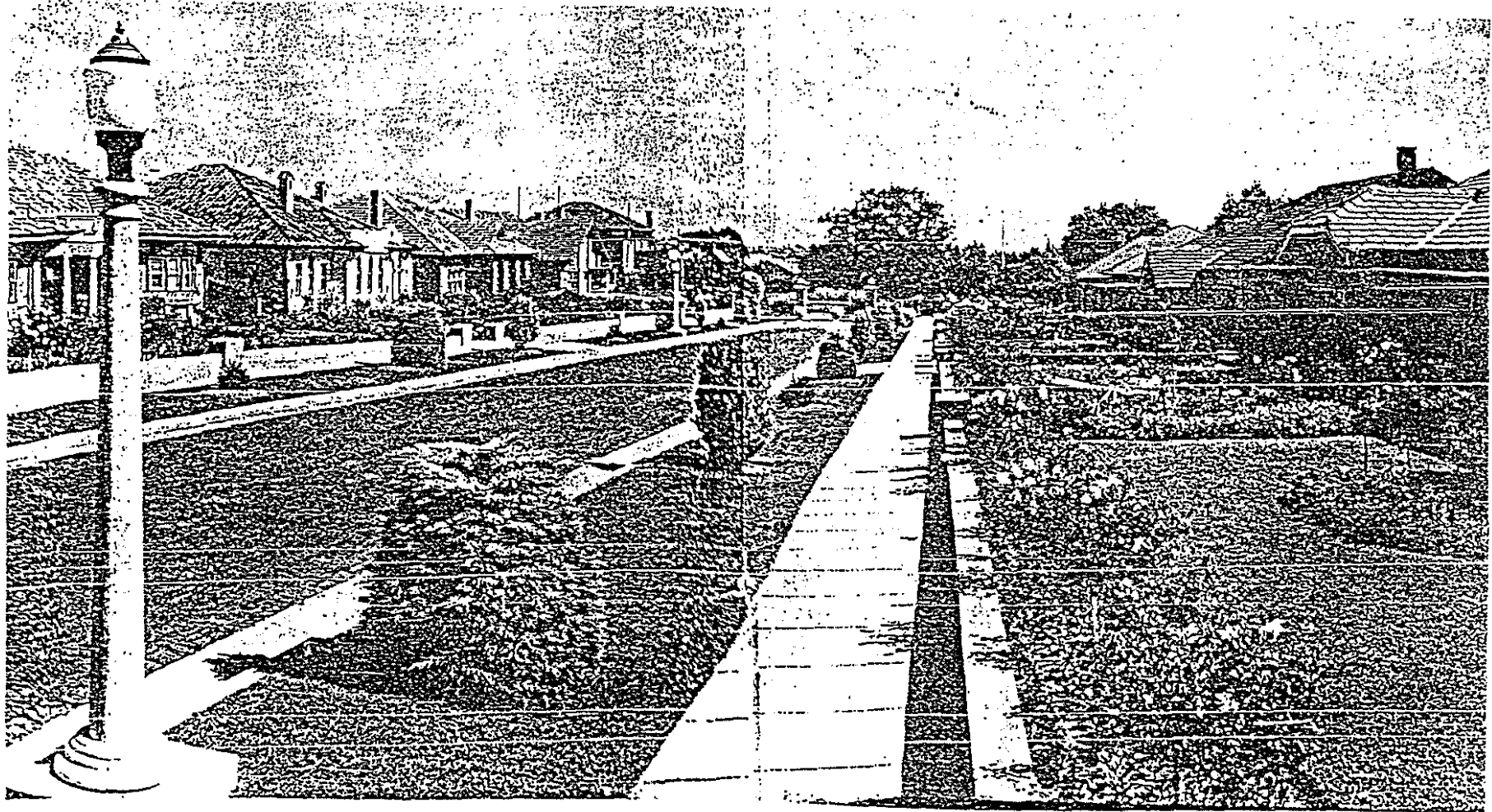
An admirable view of Lempriere Avenue, showing the advantages of lawn tips and low front and dividing fences. Note the absence of overhead wires.
