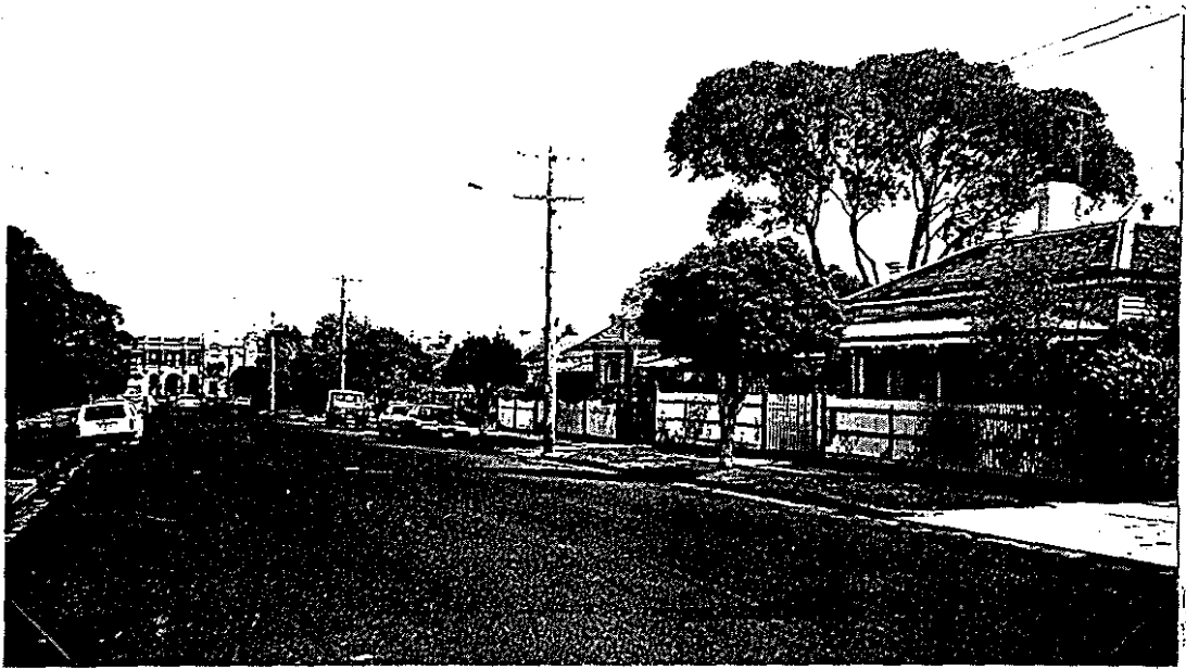
Staniland Grove, looking south to the former State Savings Bank with a row of 9 Victorian villas on the right and insubstantial street trees.
