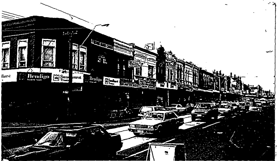
Glen Huntly Road (north side) showing the historic core between Selwyn Street and St Georges Road.
