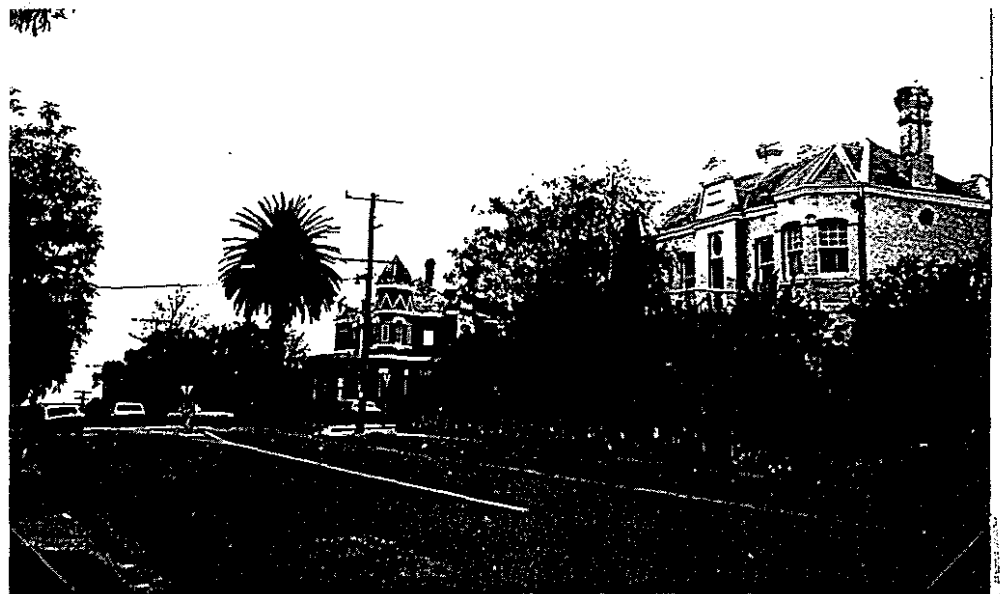
Clarence Street, looking west to the substantial Elizabethan revival villas at Gladstone Parade
