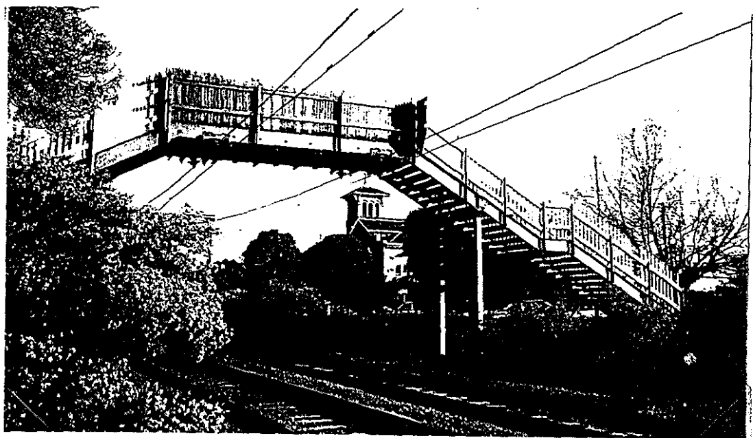
The railway footbridge, Sinclair Street.
