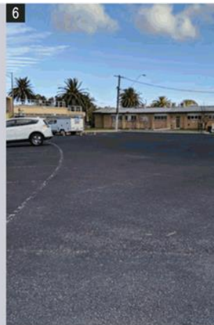
Asphalt carpark and worn line marking
