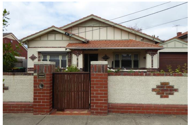
12 Rose Street, Bungalow style – gable roof
