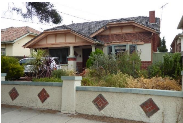
7 Rose Street, Bungalow style – hipped gable roof
