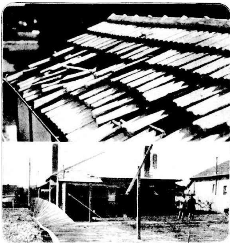
Storm damage in 1930 to roof of no. 30 and fence of no. 29 Rose Street (Source: Herald , 9 September 1930, p22)
