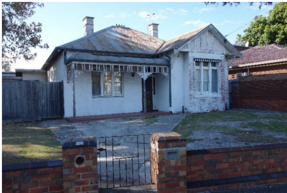
46 Grange Road – overpainted red brick, metal cresting and original/early roof cladding
