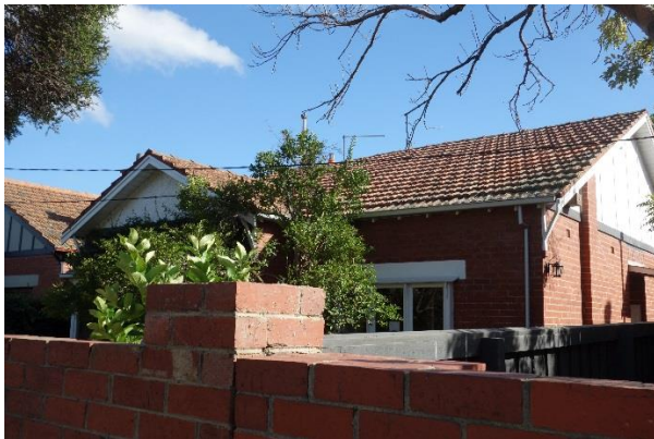
216 Neerim Road – red brick with concrete lintels
