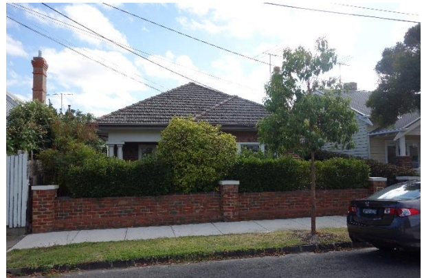
13 Edgewood Street – columns to porch and original fence
