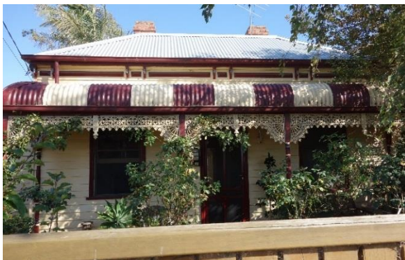
9 Byron Street – symmetrical façade, cast iron frieze and bracketed cornice
