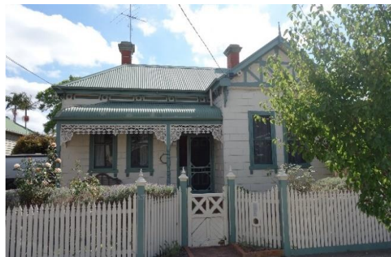
13 Hollywood Grove – cast iron frieze and bracketed cornice
