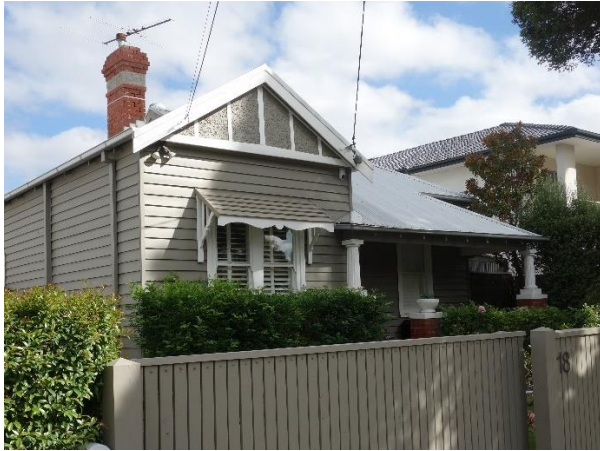
18 Mile End Road – porch with fluted columns
