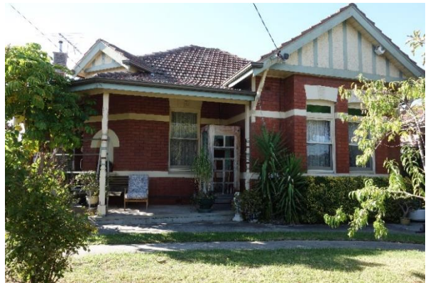
58 Grange Road – red brick with rendered bands
