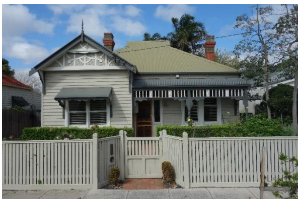
10 Holywood Grove – gambrel roof, projecting gable end and finial
