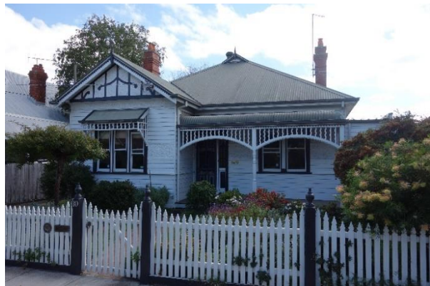
10 McPherson Avenue – varying wall treatment and arched screen to verandah
