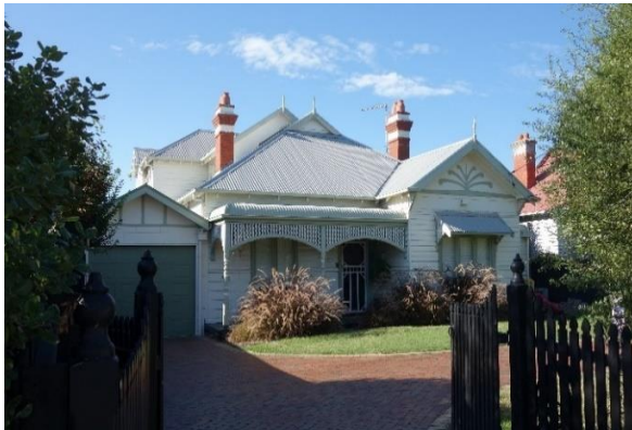
24 Grange Road – plant-like motif to gable end
