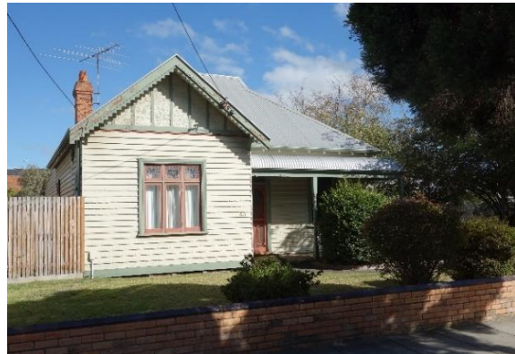
83 Mimosa Road – serrated edge to bargeboard
