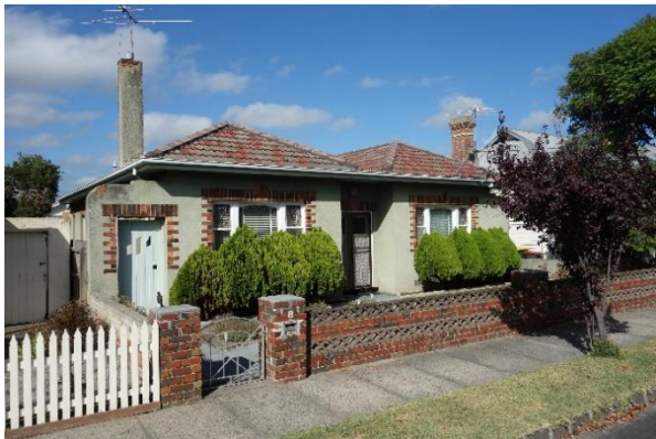
8 Edgewood Street – wall extending to boundary, original fence
