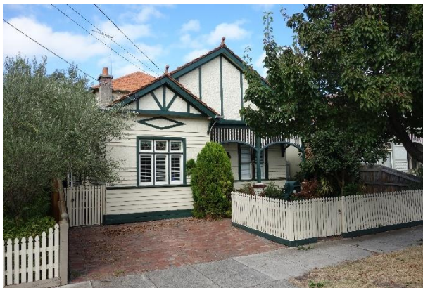
5 McPherson Avenue – late Federation example with terracotta roof tiles and shorter chimney
