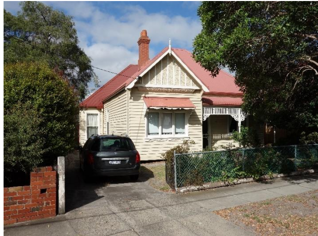
30 Munster Avenue – street roof pitch and Queen Anne sill
