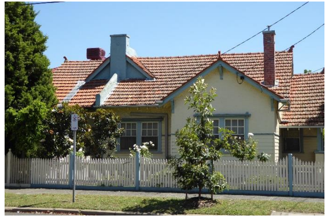
242 Neerim Road – semi-detached pair with roughcast to upper walls
