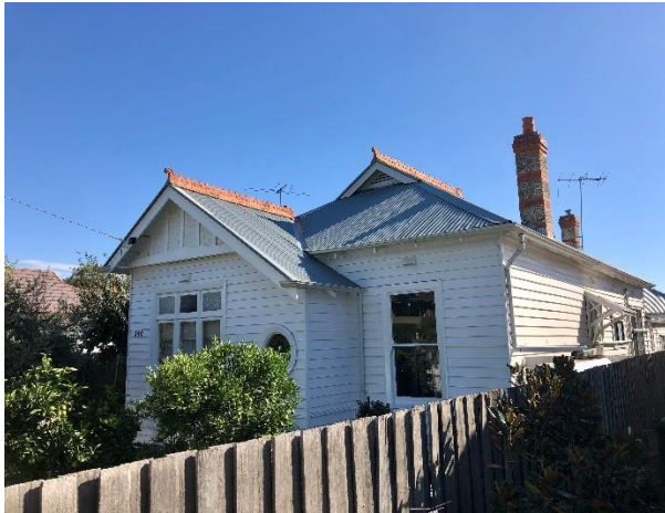
230 Neerim Road – terracotta ridge cresting, catslide roof, circular window and tall chimney with rendered bands
