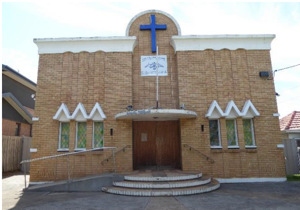
4 Gilbert Grove – church façade
