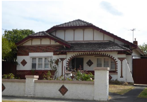
11 Campbell Street – bungalow with gable end detailing similar to some in Rose Hill Estate Precinct (e.g. nos 17 + 27 Rose Street)
