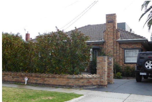
39 Burgess Street – Moderne style, late example, by 1944/45
