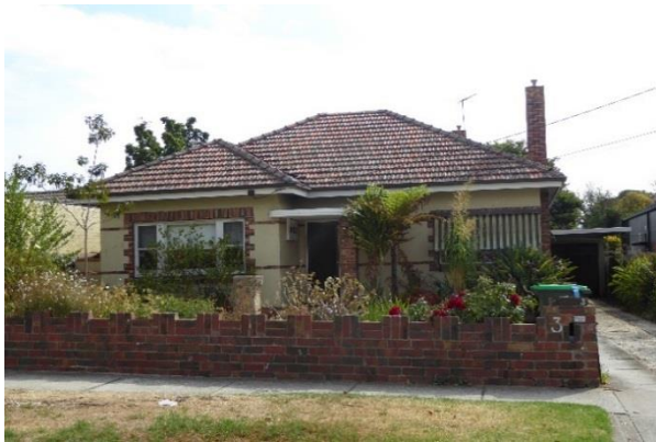
3 Burgess Street – Moderne style, late example, by 1942
