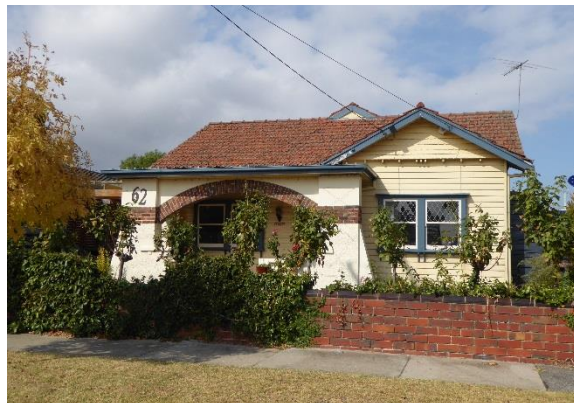
62 Mitchell Street – weatherboard bungalow with masonry porch
