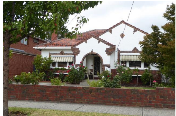
32 Gilbert Grove – Tudor Revival style with tapestry brick detailing
