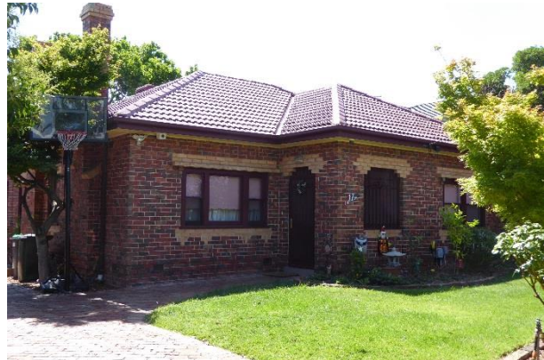
17 The Highway – corbelled openings to porch
