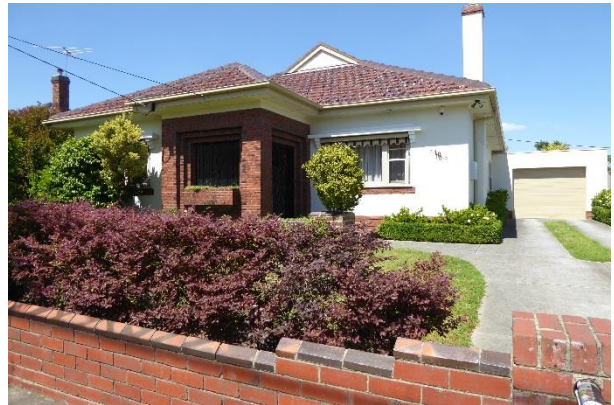
10 The Highway – tapestry bricks to porch and grass island to driveway
