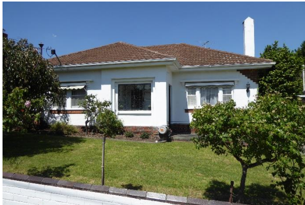
4 The Highway – stepped brickwork to corners
