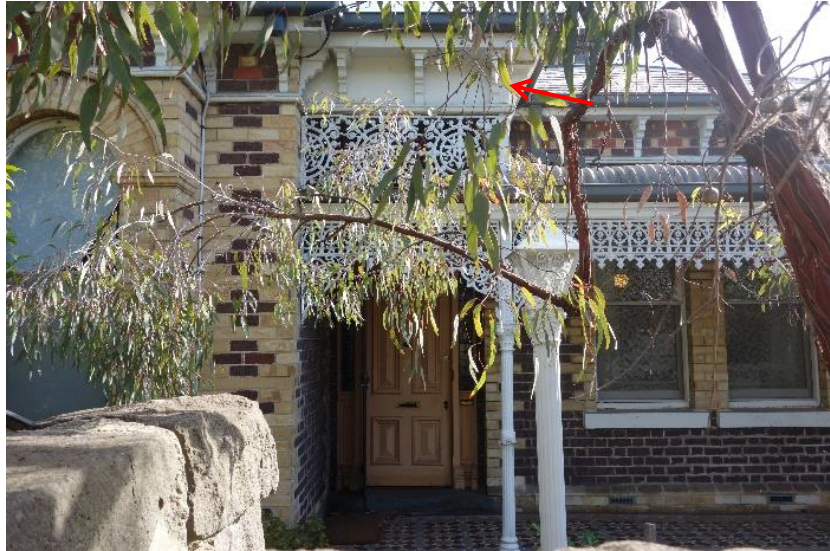
Main entry with flat-roofed entry bay indicated by the red arrow
