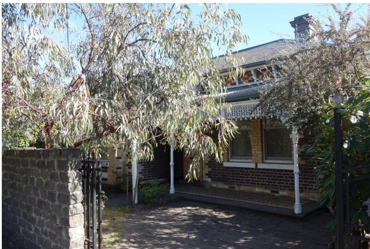
Detail of façade
