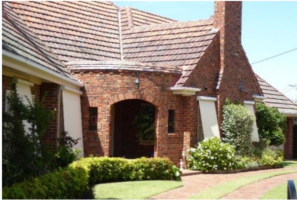
Entry portico with arched entry and gable end
