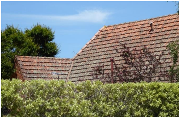
East end/rear of site
