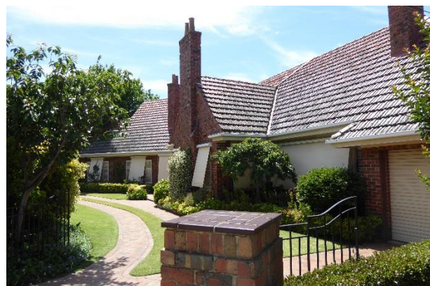
Milton Street frontage – southern end with original garage
