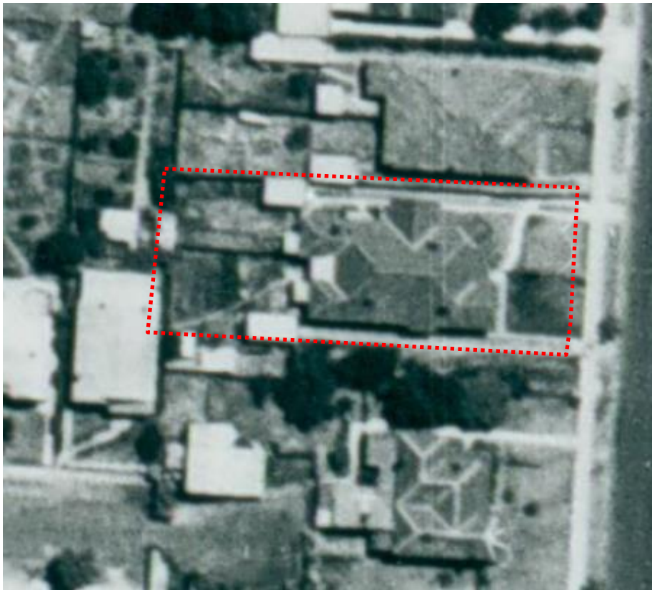
1945 aerial photograph with the subject site outlined in red and Koornang Road right of frame. (Source: Landata, Melbourne and Metropolitan Area Project, Pro. No. 5, Run 14, Frame 57711)
