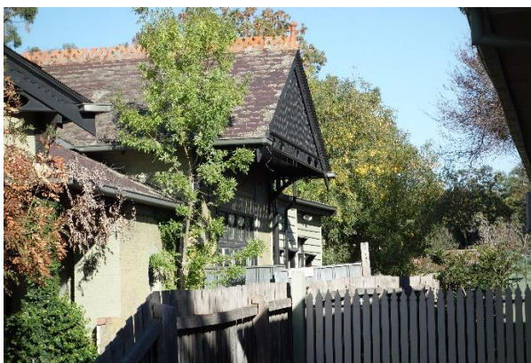
Detail of northern gable above modified bay
