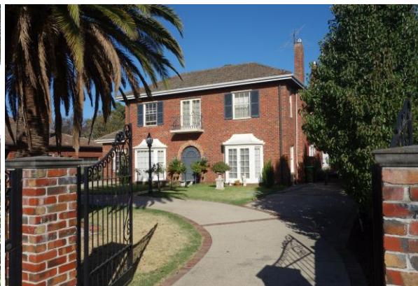
Koornang Road frontage, facing south-west
