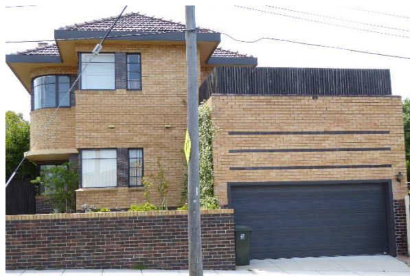
West elevation with garage
