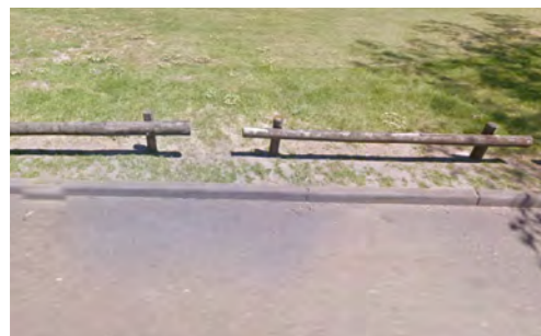
Timber Post & Rail
