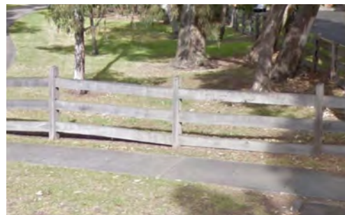
Timber P&R Fence
