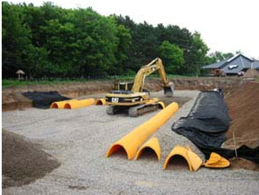
Figure 9-1 Stormtech subsurface chamber systems
