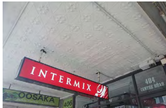
No. 404 – example of pressed metal soffit
