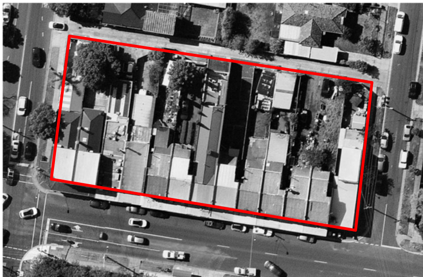
Grand View Estate Shops (red) (Source: Nearmap, 7 October 2018)
