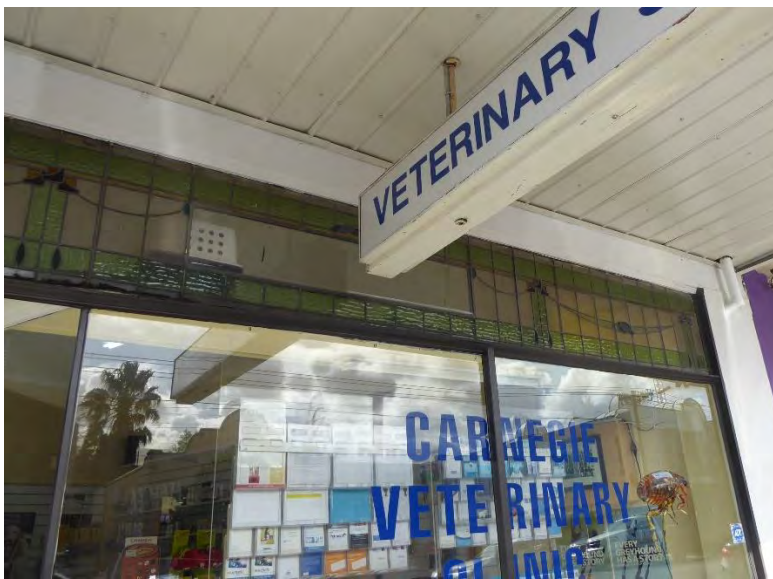
66 Rosstown Road, shopfront
