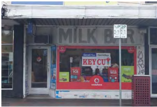
Largely intact shopfront, 247 Koornang Road
