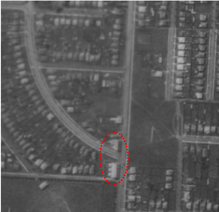
1931 Aerial, Maldon Prison Project, no.1931, run 26, frame 2474 The two groups of shops (231-237 and 241-251) are indicated (Source: Landata)
