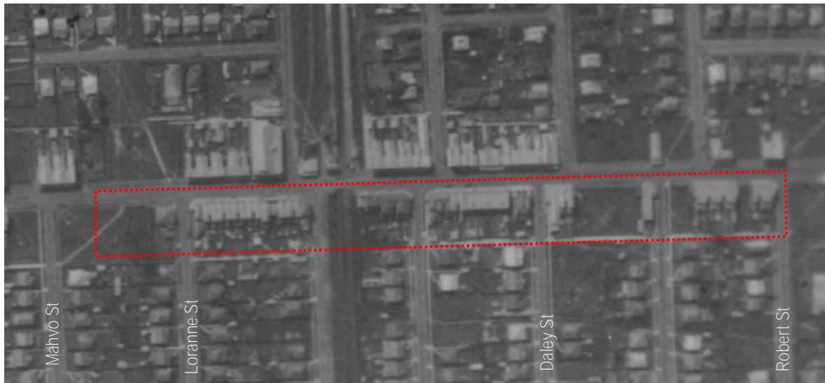
Aerial photograph dated 1931 (Source: Landata, Maldon Prison, Proj. No. 1931, Run 25, Frame 2480)
