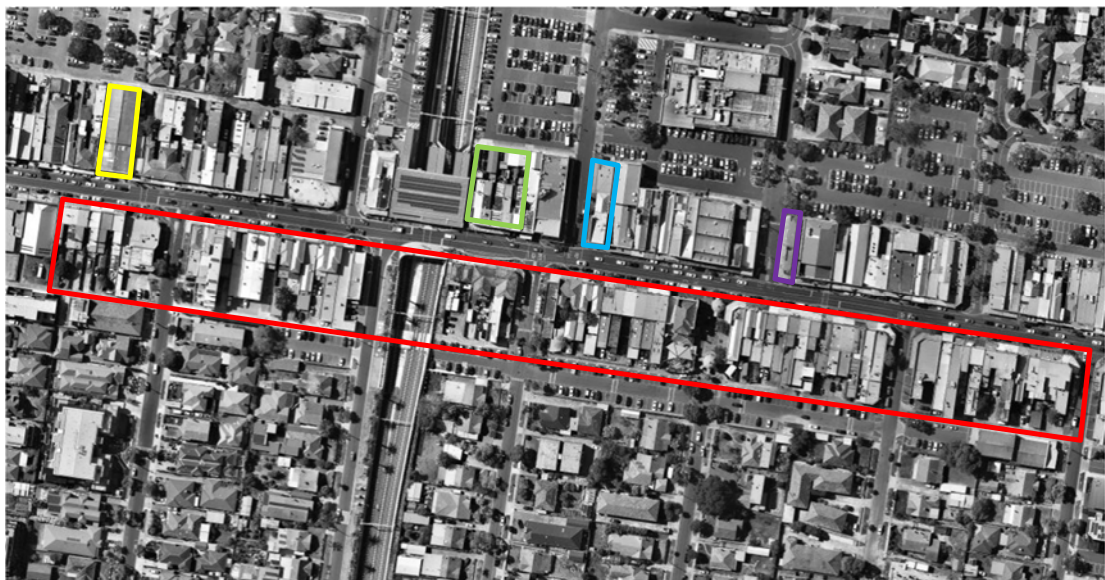
Centre Arcade (yellow) Shops, 369-377 Centre Road (green) Former ES& A Bank (blue) Former Brighton Gas Company Showrooms (purple) Bentleigh Retail Precinct (red) (Source: Nearmap, 2018)
