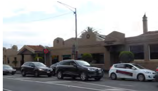
Position of former garage to the east (Koornang Road)
