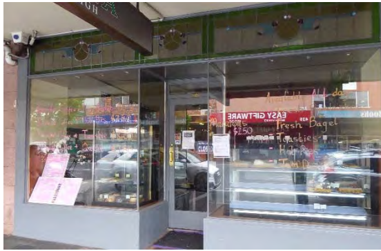
No. 482 – Interwar period shopfront with stained glass to highlights
