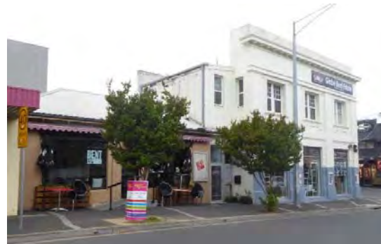
West elevation (Bent Street) – south end
