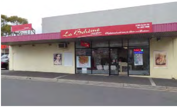
West elevation (Bent Street) – north end
