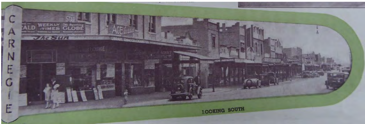
1938, West side of Koornang Road (north of Neerim Road) (Source: Auction Notice, Glen Huntly Park Estate, Glen Eira Historical Society)
