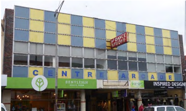
Centre Road, Bentleigh
