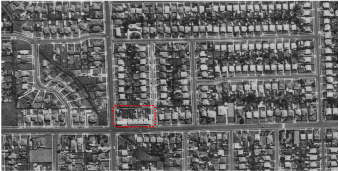
1956 aerial photograph. The subject shops are indicated (Source: Landata, Melbourne Outer Suburbs Project, no. 250, run 28, frame 99)
