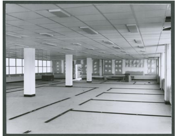
Interior of stage 4 administration building
