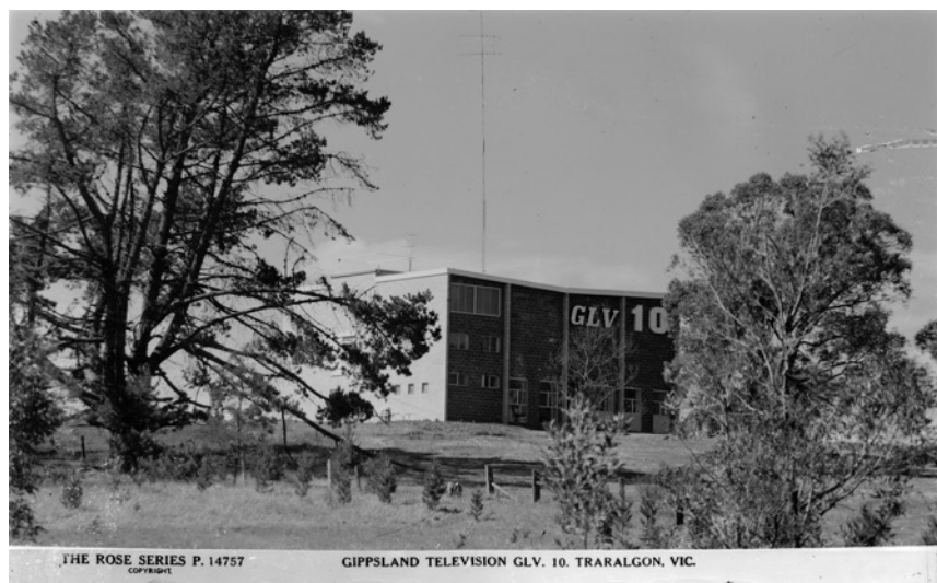
GLV10 Traralgon opened December 1961. Source, SLV
