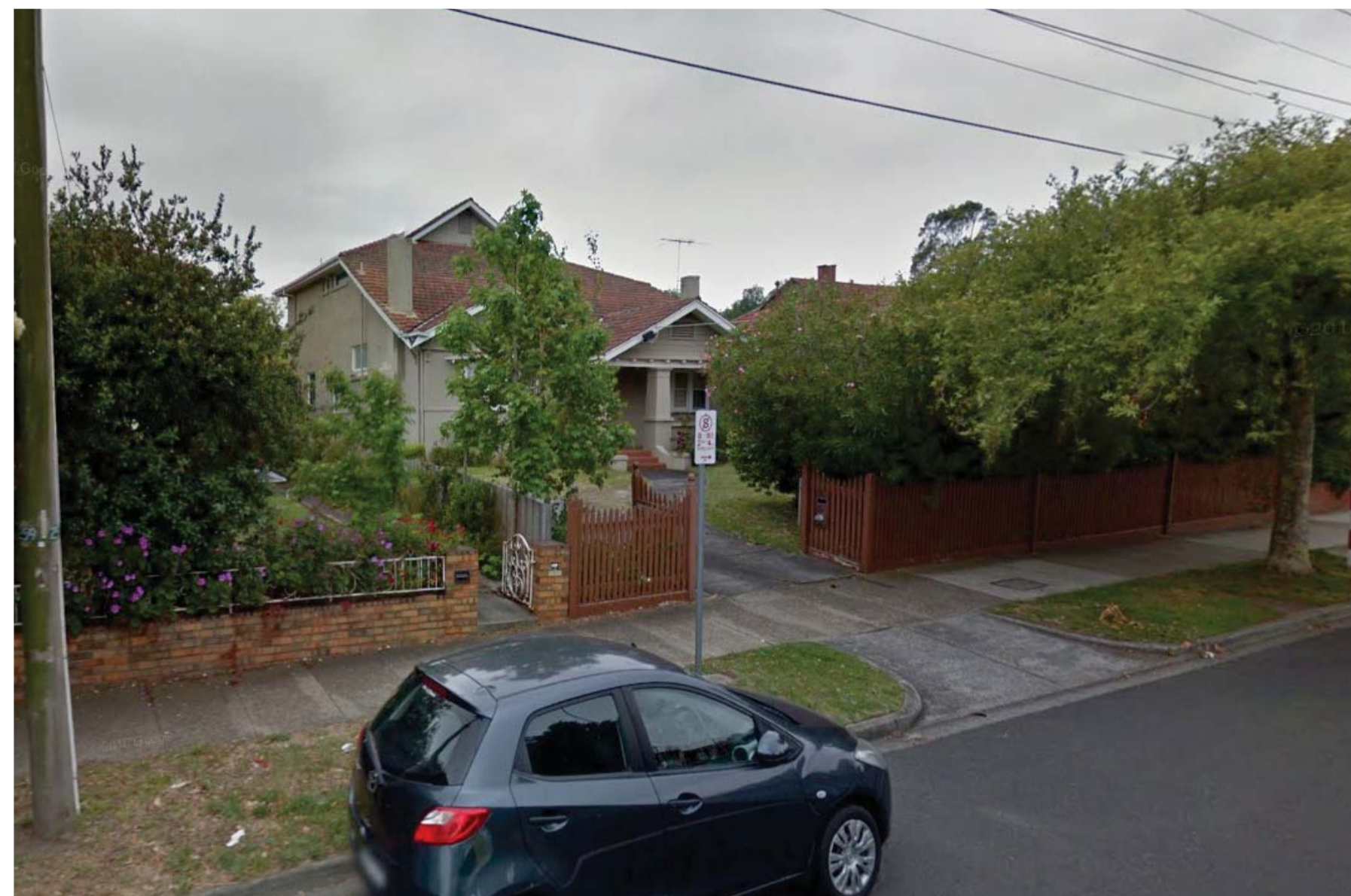
1 - View of 259 and 261 Glen Eira Road
