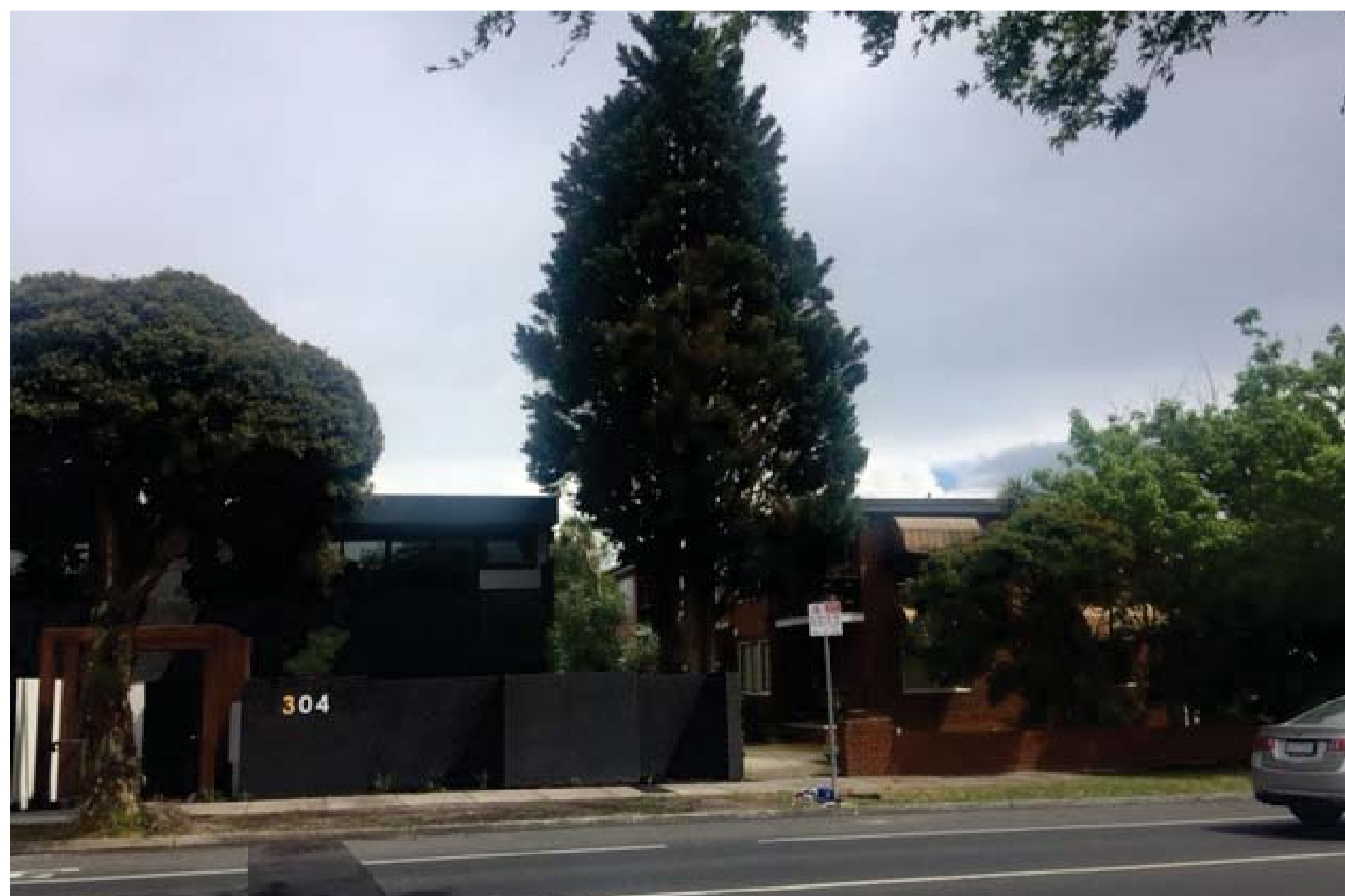
6 - View of 304 and 302 Glen Eira Road
