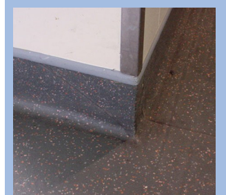
Vinyl sheeting floor with coving.
