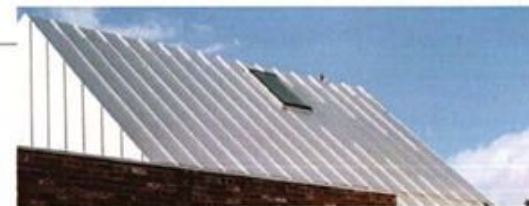
CL04 - STANDING SEAM CLADDING COLORBOND - SURFMYST
