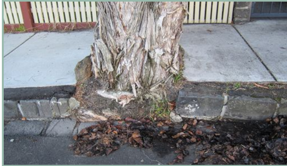
Figure 07. Example of Melaleuca outgrowing a standard planting pit in Prentices st. Elsternwick.
