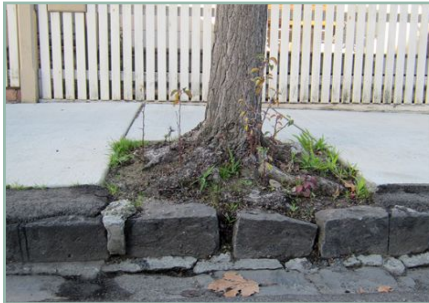
Figure 03,04,05. Example of another Pyrus located within Edward st, Elsternwick that has outgrown the original planting pit and damaged the footpath has been replaced. New cracks and further lifting of concrete is occurring.
