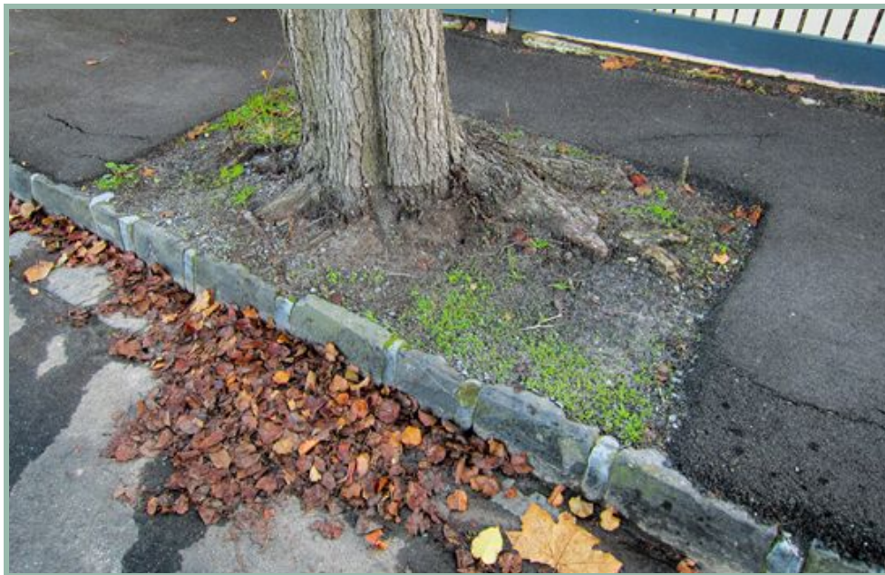
Figure 01,02. Example of a Pyrus located within Edward st, Elsternwick that has outgrown the original planting pit and damaged the footpath to the extent that the concrete has been replaced with asphalt. The cracks in the new asphalt indicate an active root system high in the soil profile. This species is the selected species for the street.
