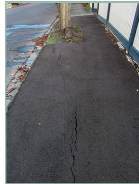
Figure 01,02. Example of a Pyrus located within Edward st, Elsternwick that has outgrown the original planting pit and damaged the footpath to the extent that the concrete has been replaced with asphalt. The cracks in the new asphalt indicate an active root system high in the soil profile. This species is the selected species for the street.
