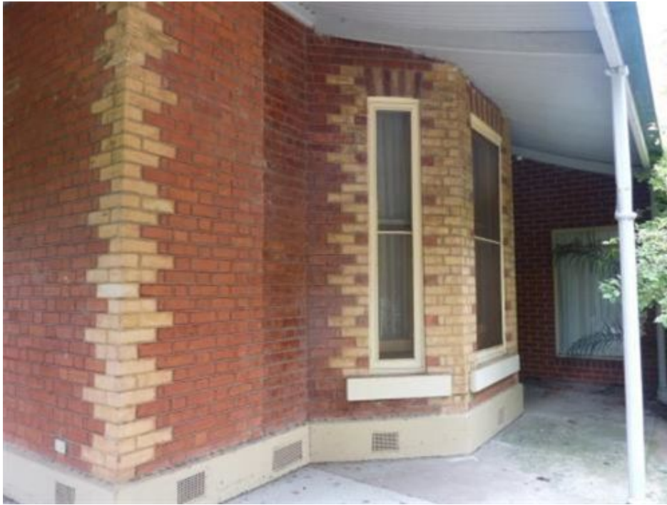
Detail of polygonal bay and polychromatic brickwork.
