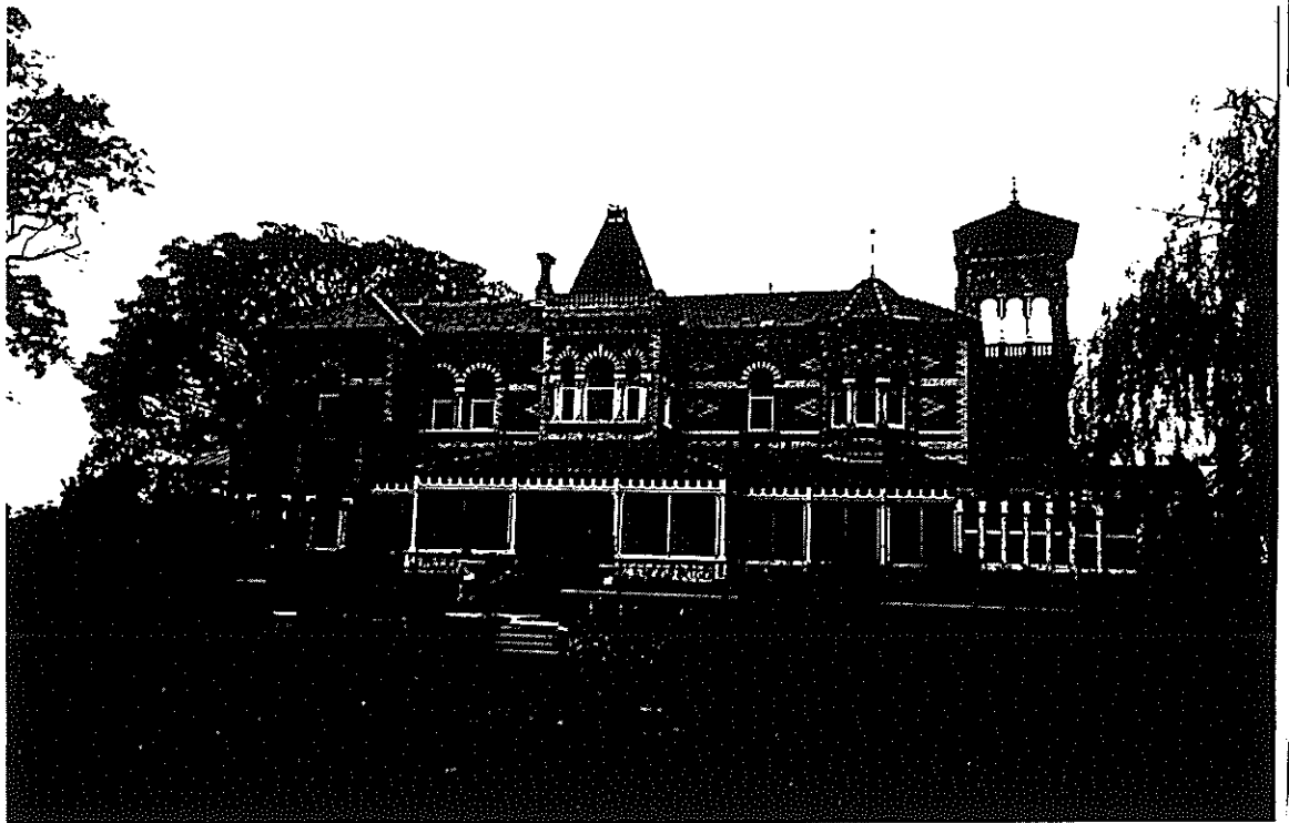
West elevation (facade)
