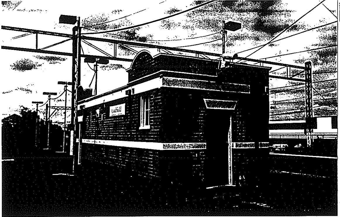
Stores building: Platforms 2 and 3
