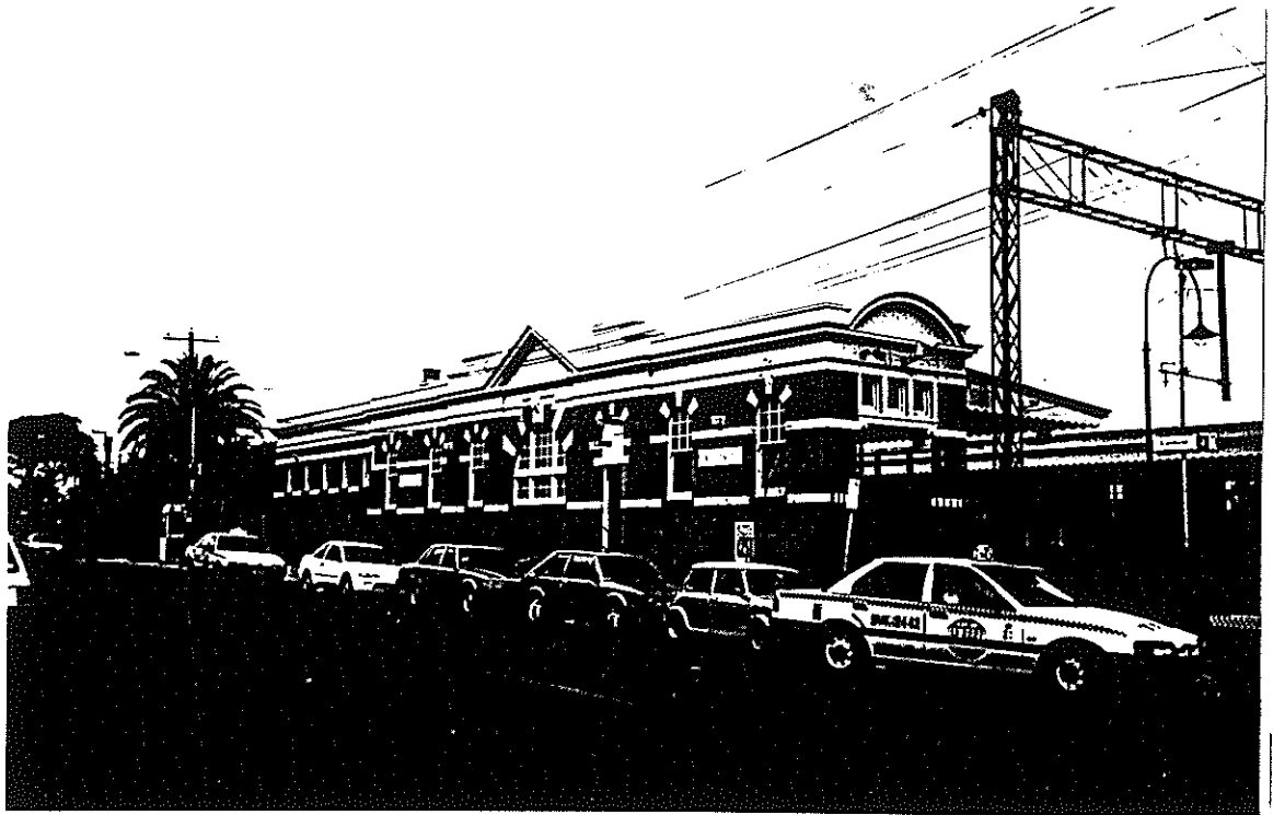
Platform 4 building: Railway Avenue
