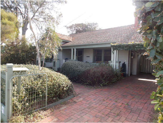
Figure 5: Timber bungalow at No 13 (1925; one of the first houses in Field Street)
