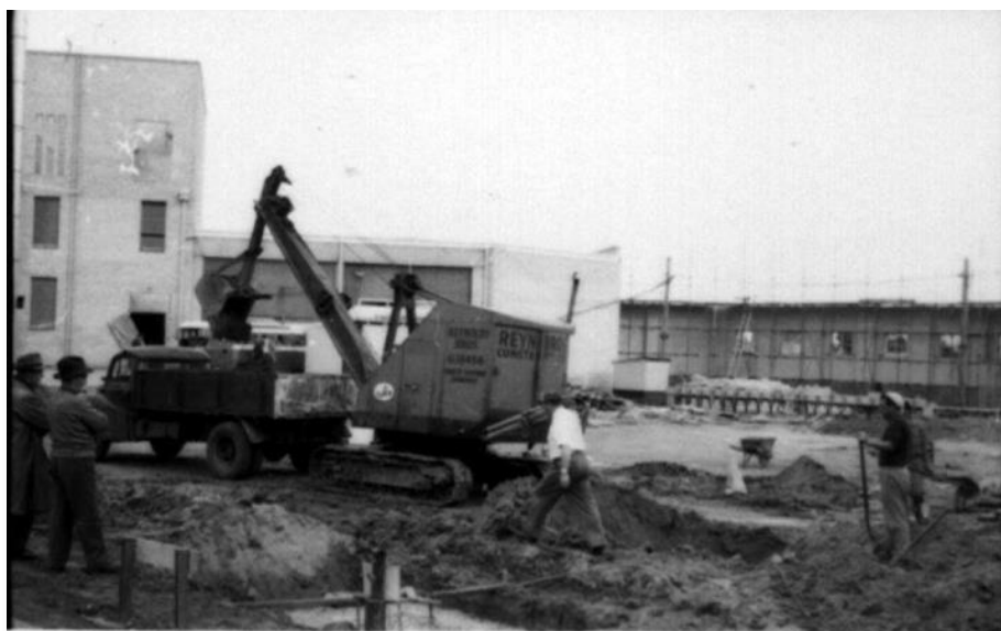
Site excavation of studio building circa 1956. This is construction of stage 2 of the Ripponlea facility with the scenery workshop wall along the railway in the course of construction at the rear. Source www.abv2.net.au
