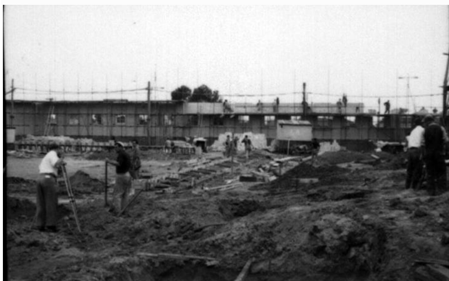
Studio building excavations for Stage 2, (footings of major studios) with scenery workshop wall in place at rear, circa 1956. Source, http://www.abv2.net.au/
