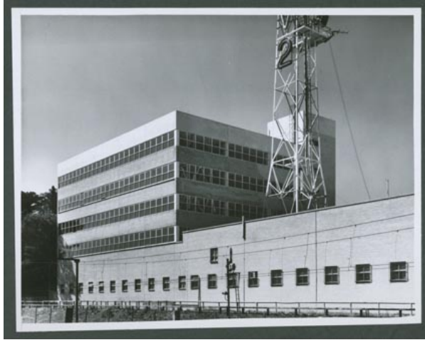
Four storey administration building in course of being finalised in 1968, view to north-east along rail line.
