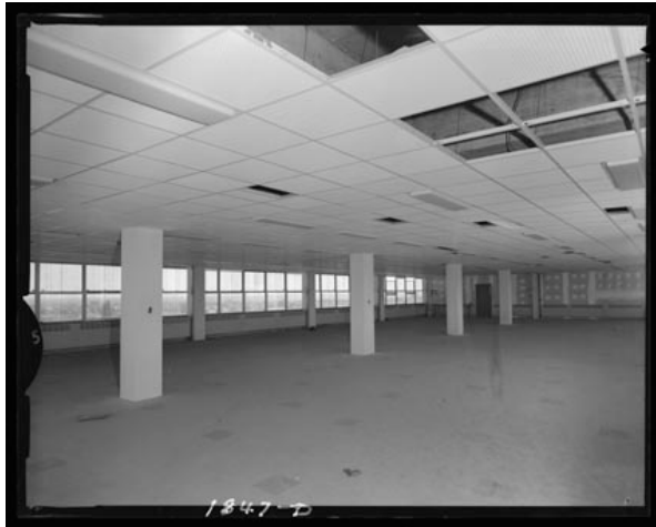
Interior of stage 4 administration building with gridded drop ceilings, concrete encased columns, strip windows, vinyl floor finish over concrete.
