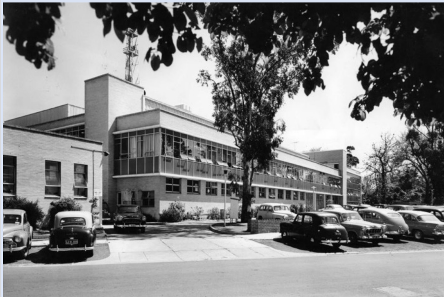
ABV 2 offices from Gordon Street, circa.1961. Source, www.ABV2.net.au
