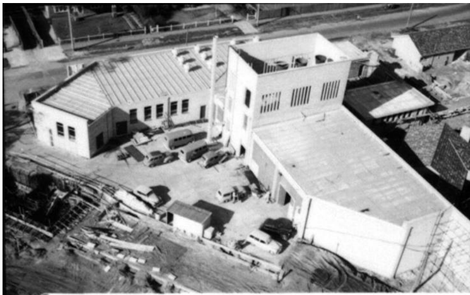
Emergency generator area (within 3 storey building) and outside broadcast garage from the transmission tower, circa 1956. This is Stage 1 of the Ripponlea facility. Source www.abv2.net.au
