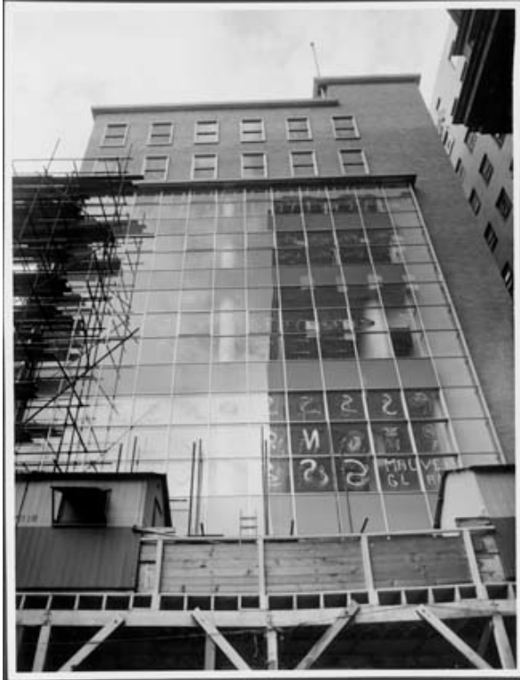
The Russell Street Telephone Exchange building at 376-382 Flinders Lane, Melbourne, commissioned by the Commonwealth Department of Works and built by Clements Langford in 1956-7. National Archives Australia: B6295, 260C
