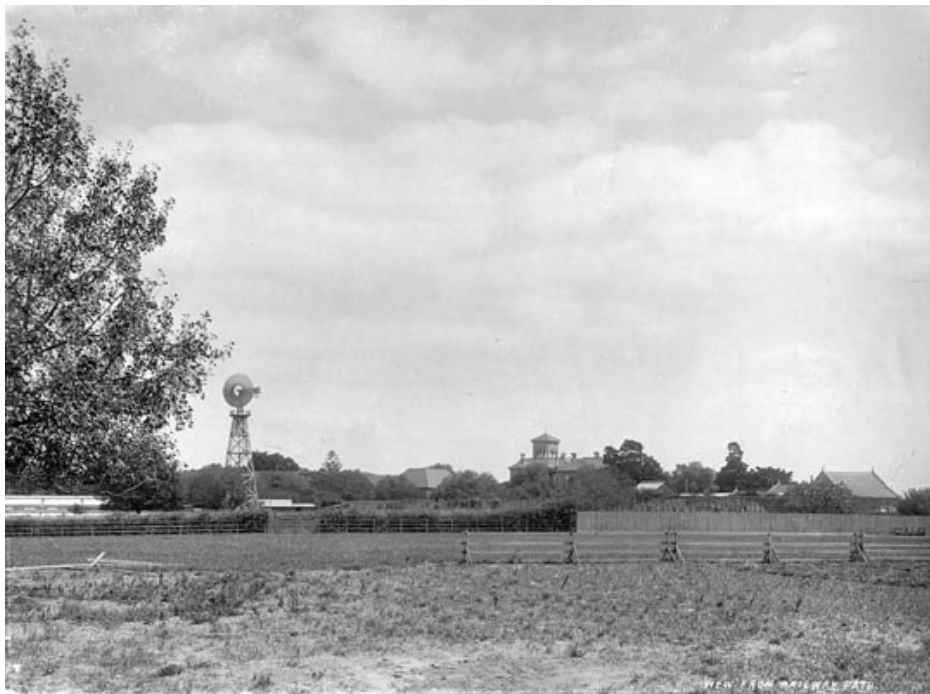
View from Railway Path, looking back toward Rippon Lea, 1903 ( in the paddock area where the ABC building was later developed). Source, Johnstone, O'Shannessy & Co. photographers, SLV
