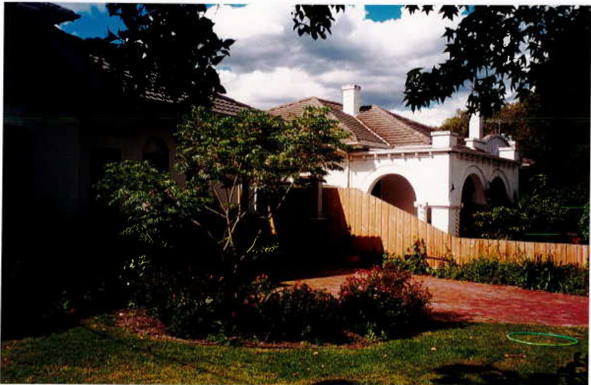
North side villas, showing the low side boundary fences between allotments
