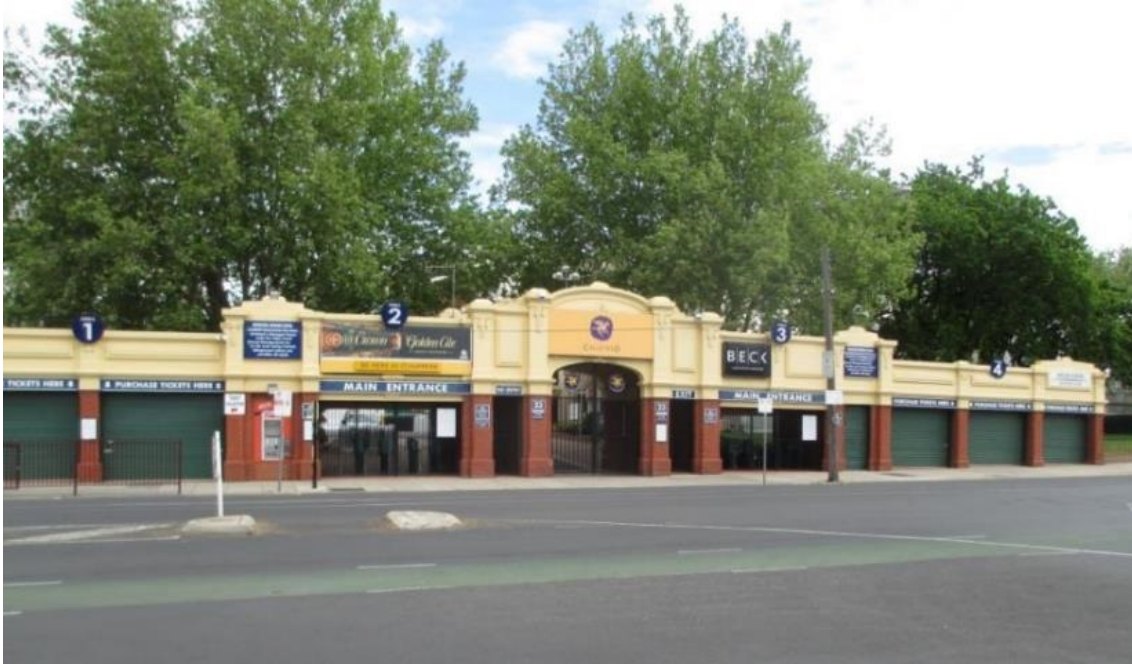
Figure 7 Gatehouse to Station Street
