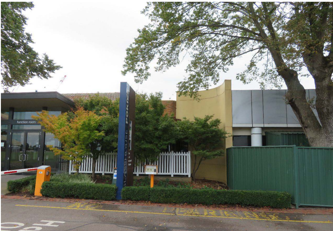
Figure 14 View of the south façade of the Afternoon Tea Room, showing Glasshouse addition to the east
